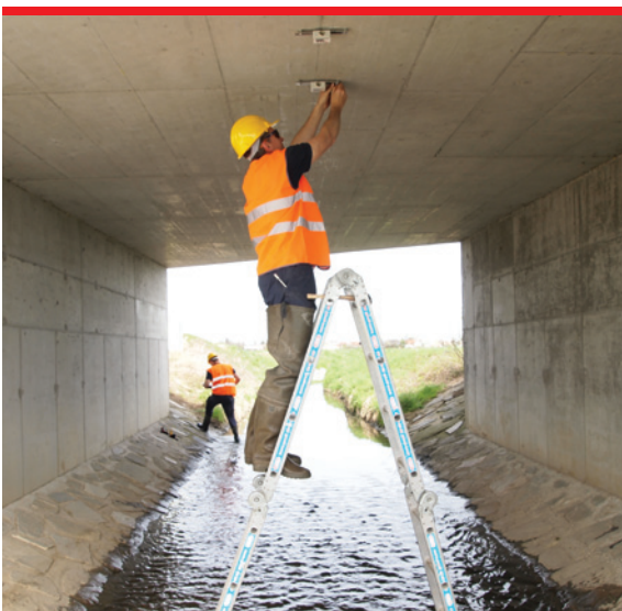
Set up of the sensors under slab bridge.
