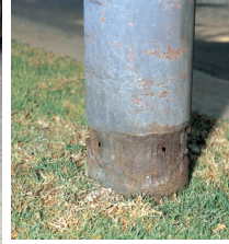
Corrosion of steel pole
